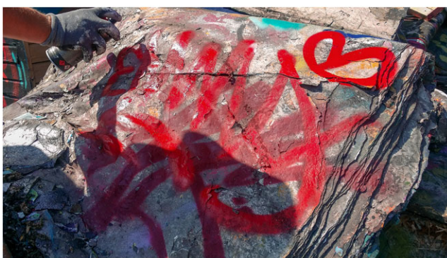
FIGURE 8 A graffiti artist at Gamlebyen Skatepark paints over thousands of layers of accumulated spray paint that collapsed a wall (2016)
